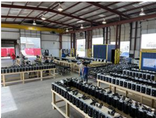
Odessa Data Center Staging Area
