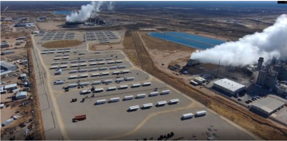
Odessa Data Center Area B & C
