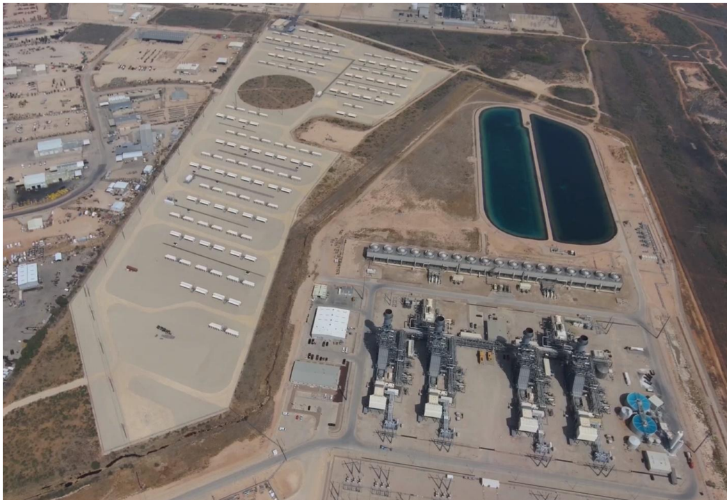
Cipher Mining's Odessa Facility
