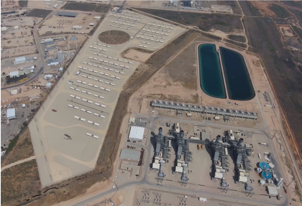
Cipher Mining's Odessa Facility
