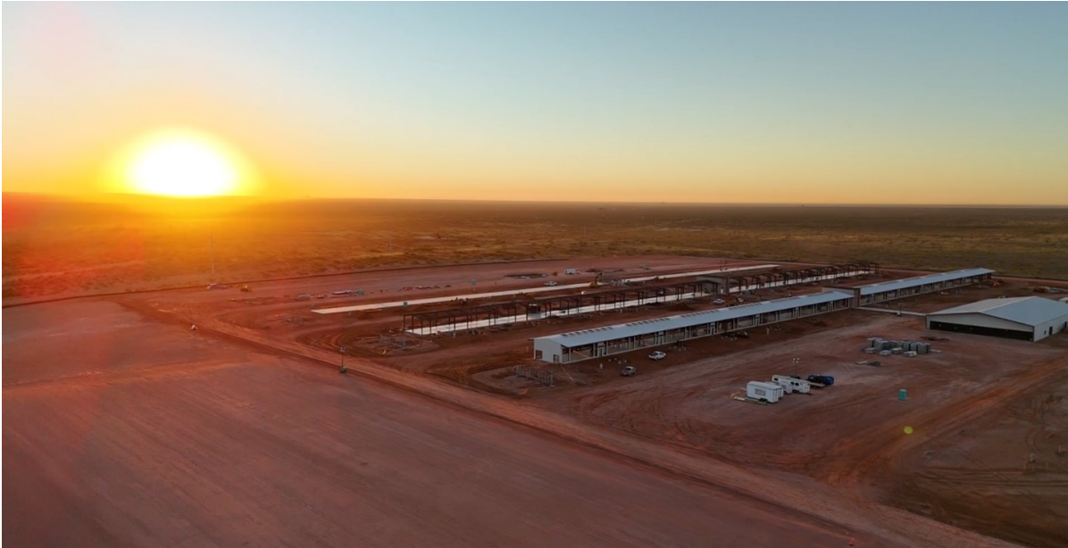
Construction at Black Pearl Site
