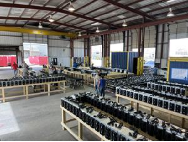
• Odessa Data Center Staging Area
